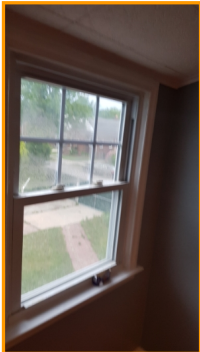
Replace cracked panes
