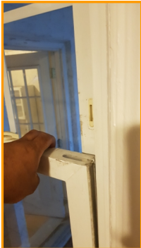
Damaged tilt locks
