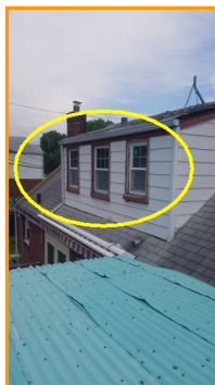
Replace damaged wood trim
